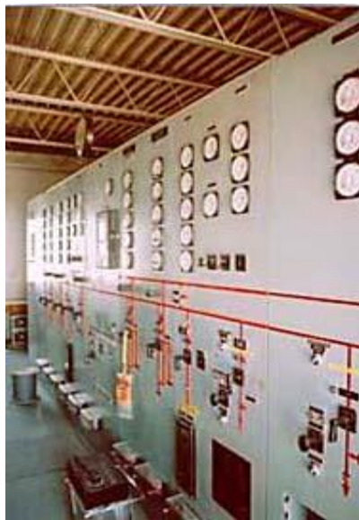
Figure 1. Substation control panel
