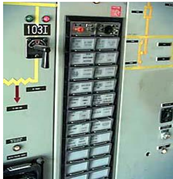
Figure 2. Substation control panel, detail
