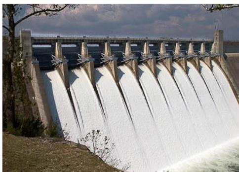
This is the normal reservoir level. If a flood enters the reservoir at this time, the water level will start going up and simultaneously water will start flowing out through the spillway. The rise in water level in the reservoir will continue for some time and so will the discharge over the spillway. After reaching a maximum, the
