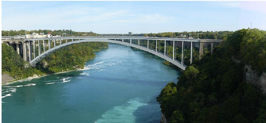
(c) A parabolic arch bridge (The parabolic arch is in compression)
