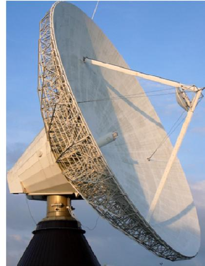
(b) A parabolic antenna
