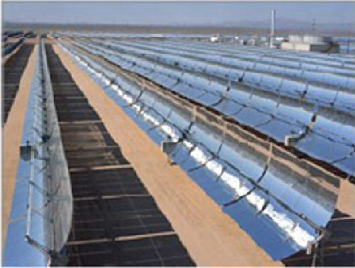
(a) An array of parabolic troughs to collect solar energy
